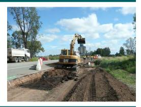
The \$7.5 million Burnett Highway (Hodgetts to Argoon Roads) Project is situated between Dululu and Biloela. This project includes the widening of approximately 8.7 kilometres of the highway to a 9 metre seal, culvert extension, property access upgrades and intersection improvement works.
